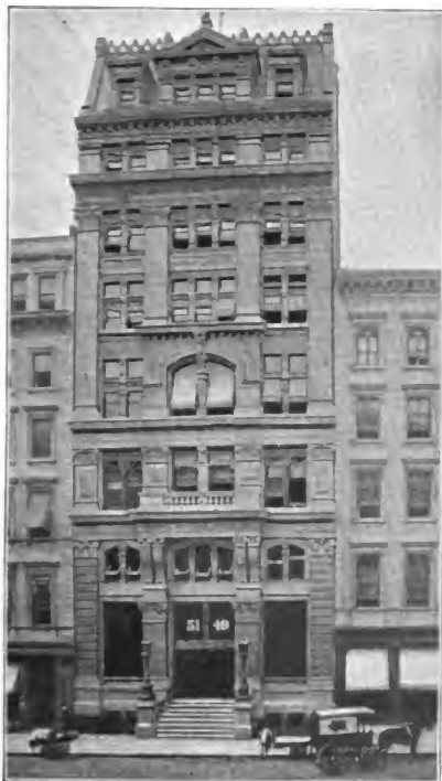
EMIGRANT INDUSTRIAL SAVINGS-BANK, 49 AND 51 CHAMBERS STREET.
